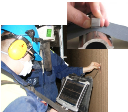
Figure 3. Probes are profiled to match the boiler tube, then connected to the ultrasonic testing equipment for accurate measurement.
